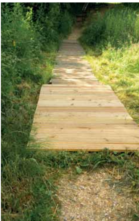
Starting to repair the board walk.
